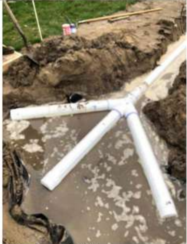
Homeowner's images of installing footing drainage from May 5, 2019.
