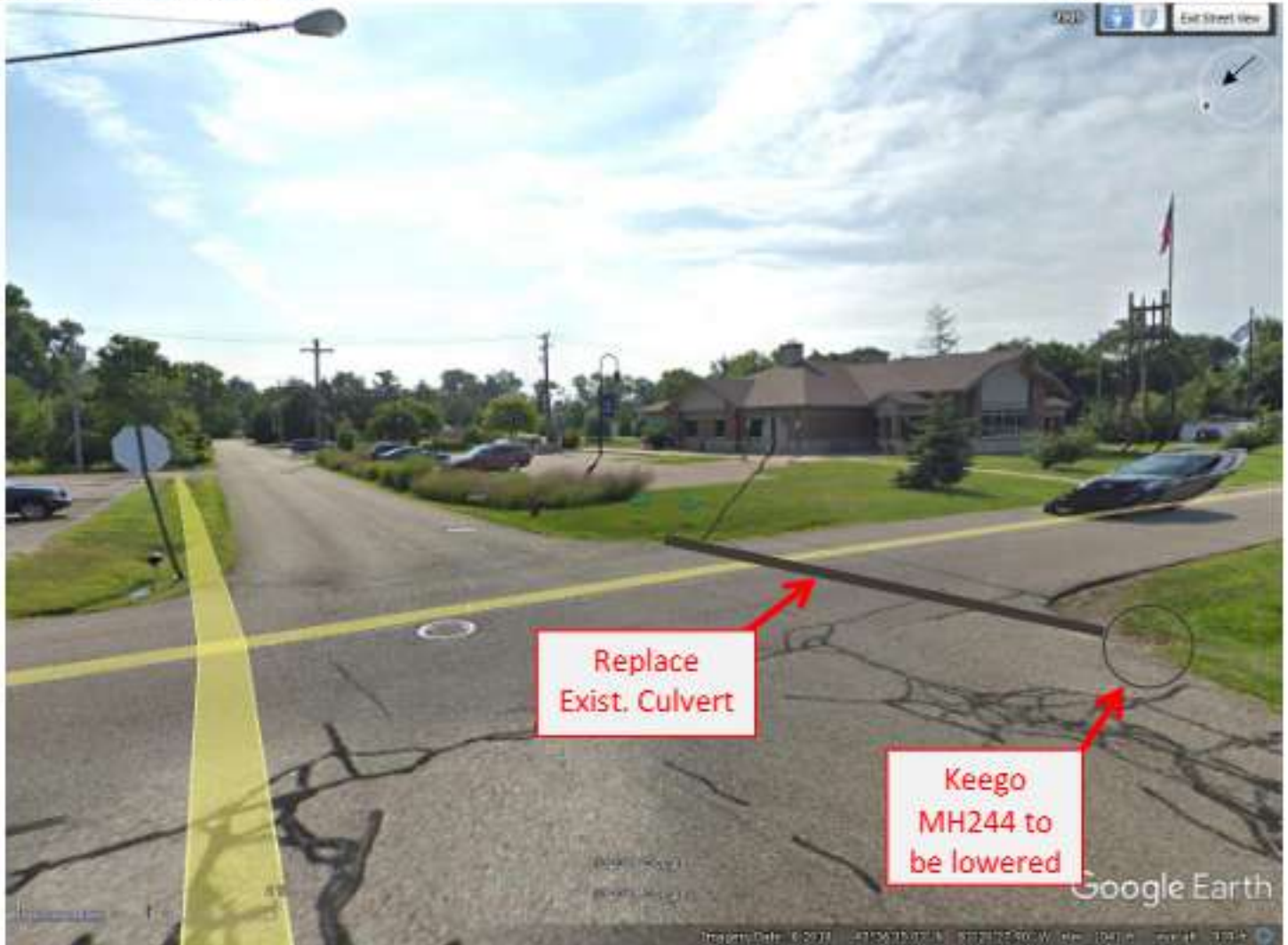
Google street view image taken in August 2018 of Schroeder Blvd., facing east and showing the location of the repair recommendations to existing manhole and culvert.
