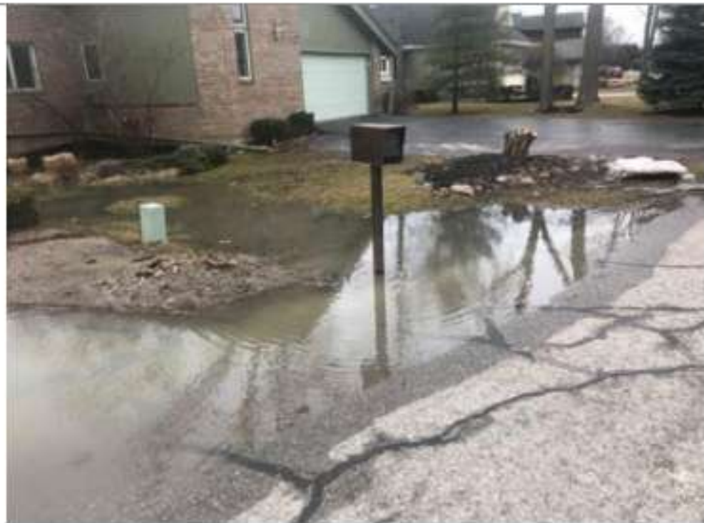
Homeowner's images of flooding in their driveway from May 7, 2019.
