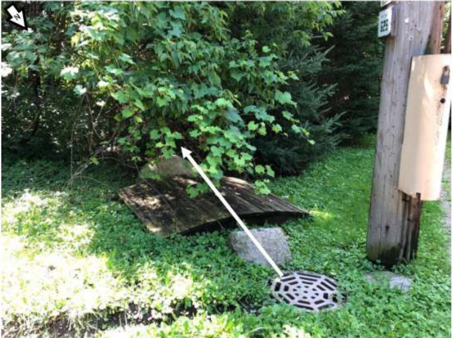
Location of the manhole at the end of Maddy Ln that discharges to the stream.
