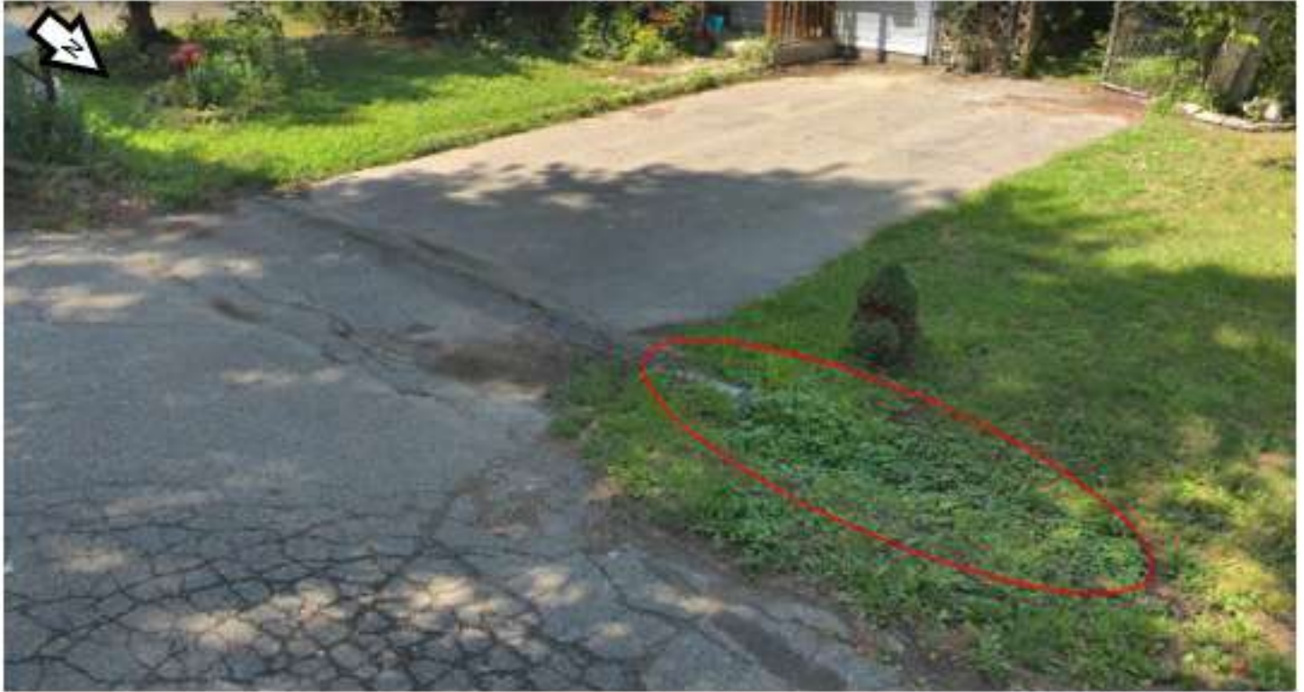
Buried culvert and ditches.
